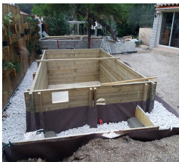
PROFIL DOUBLE RAINURE 58 X 130 MM
